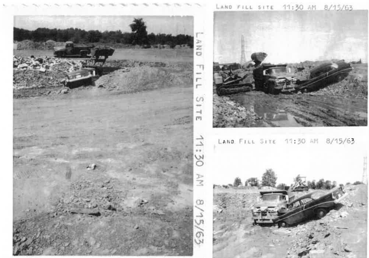
Figure 4: fotos of landfill in operation dated August 15th, 1963
